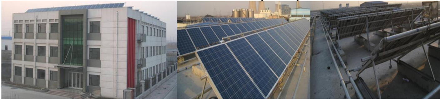
Net Zero Energy Consumption Complex Building in Dongying City Shandong Province, China (2000 m 2 )
